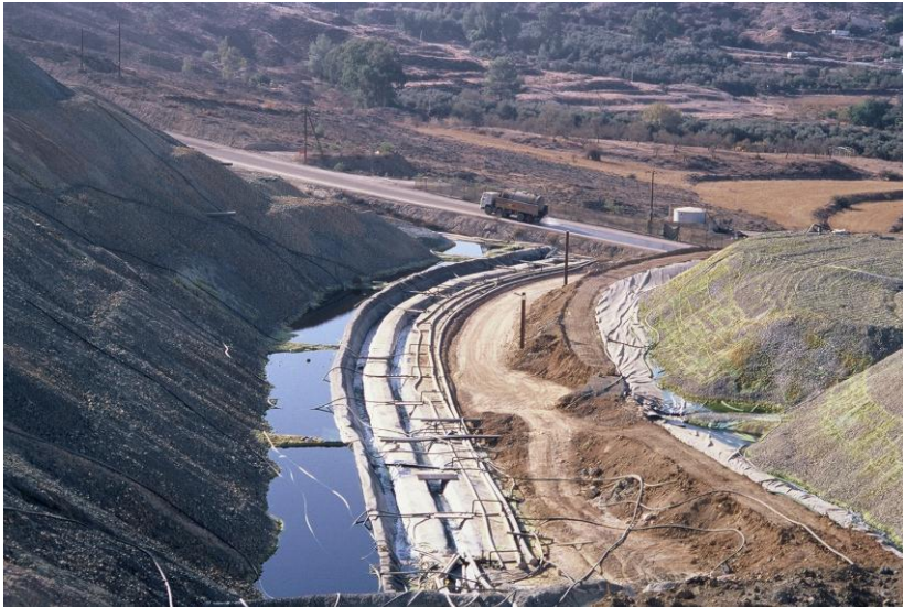
Liquid Copper transferred from Heap Leaching to PLS- ILS ponds
